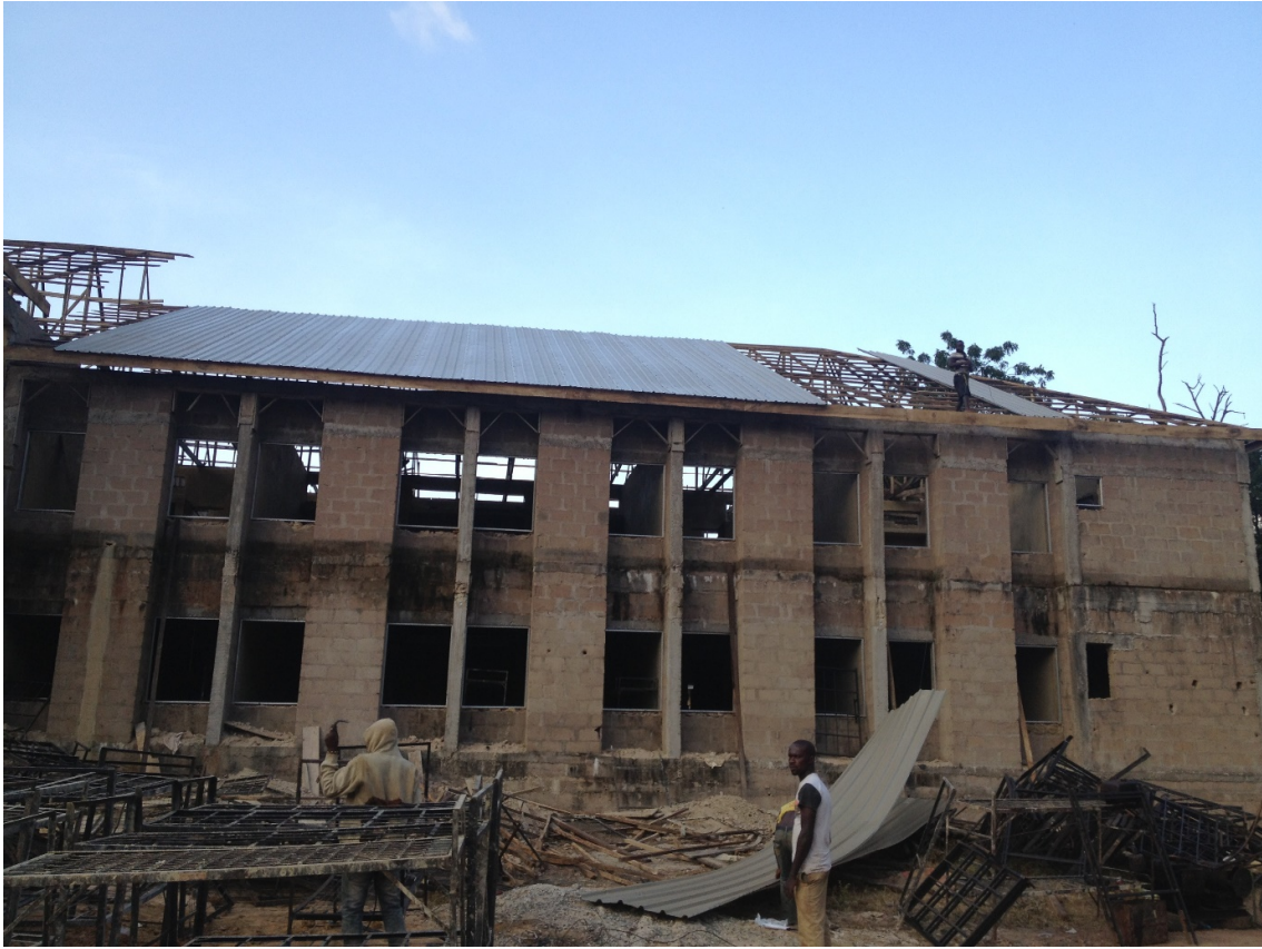
Fig. 2.4. 40 Room Hostel at NYSC Camp under Construction
