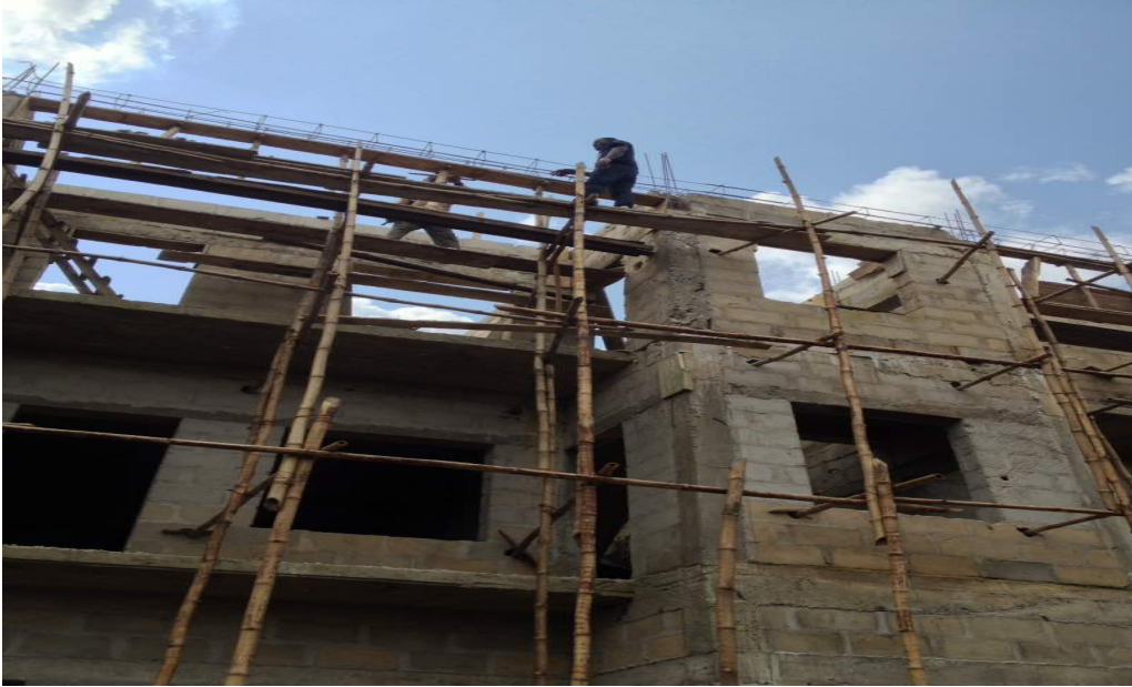
Fig. 2.2. Mr. Aneke's House under Construction
