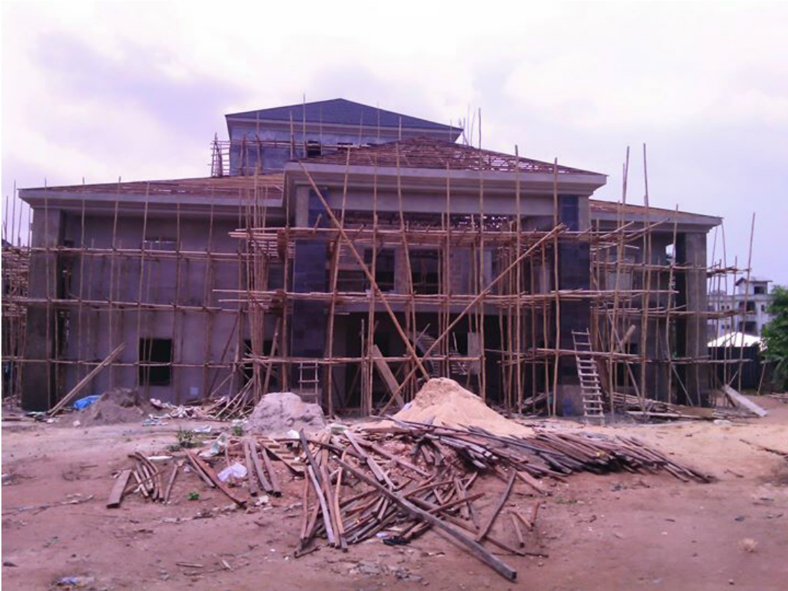
Fig. 2. 6. Six Bedroom Duplex for Mr. Ozoh under Construction
