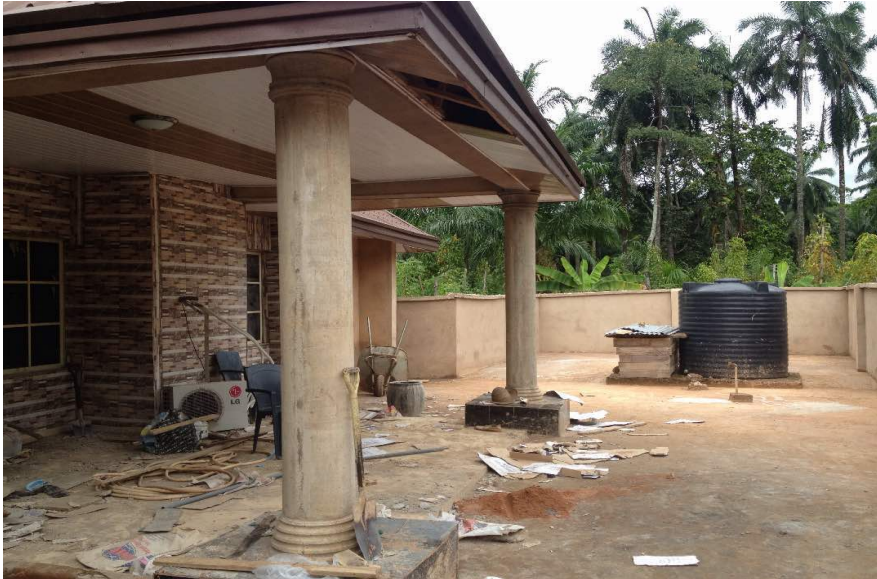
Fig. 2.3. Mr. Augustine's Bungalow under Construction
